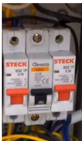
Figura12. Interruptores Termomagneticos
